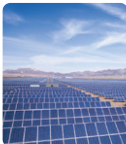
Solar/wind energy storage system
